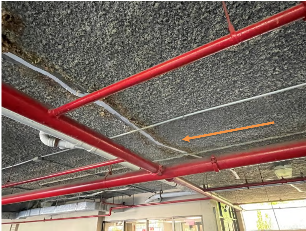
Figure 47 – Repair in progress on parking garage ceiling
