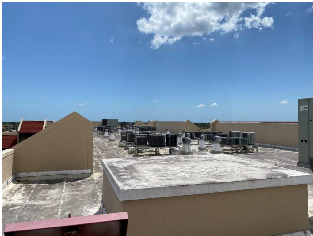
Figure 21 – Upgraded A/C stands
