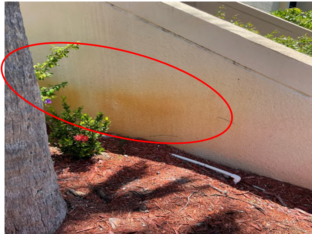
Figure 29 – Paint discoloration due to constant water exposure
