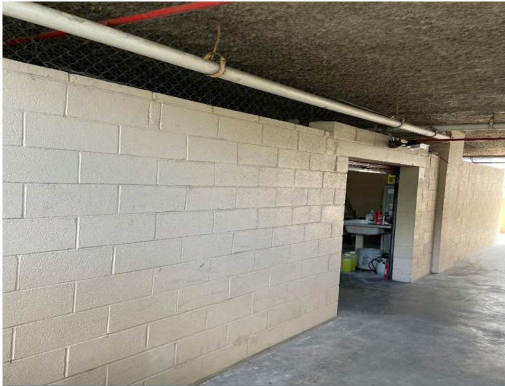
Figure 11 – Typical CMU wall found in parking garage
