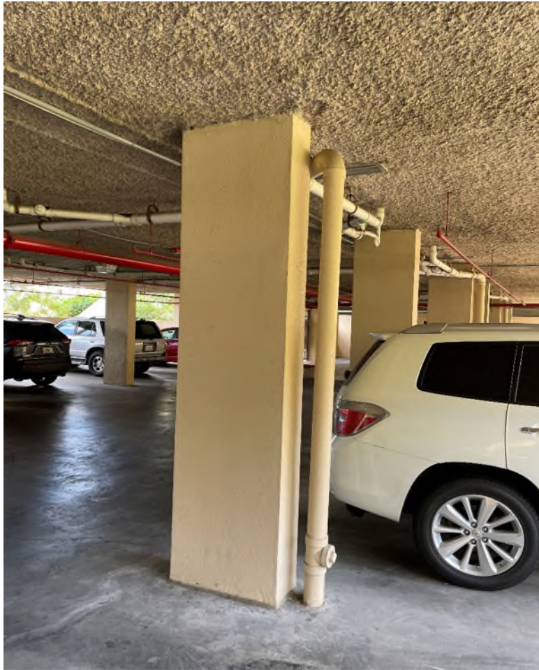
Figure 6 – Typical column found in the parking garage
