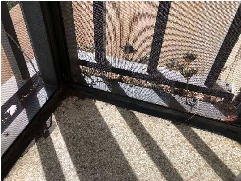
Figure 39 – Plant growth on balcony deck and through railing system - Unit 226
