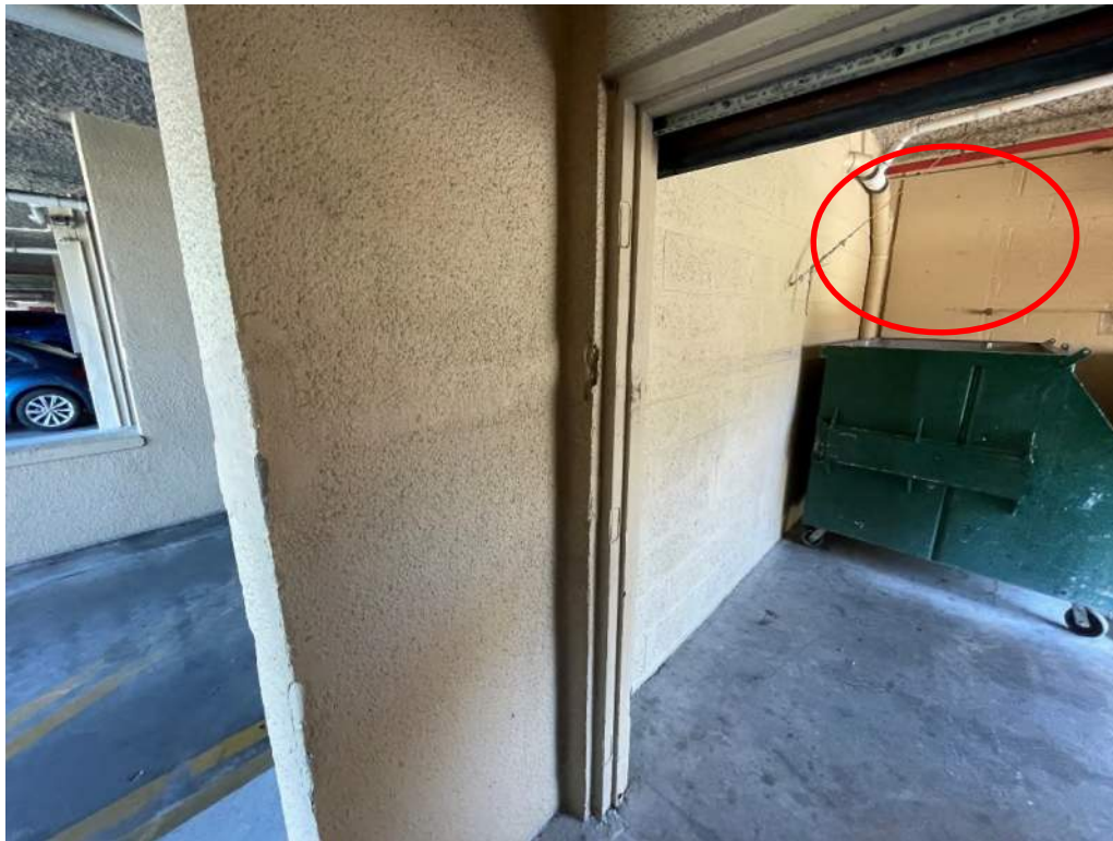
Figure 15 – Typical column located in the Trash room
