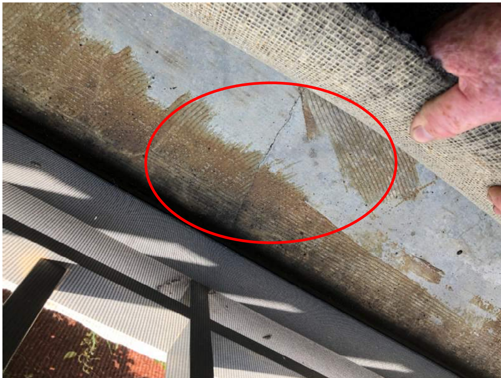
Figure 41 – Typical crack in balcony slab - Unit 214
