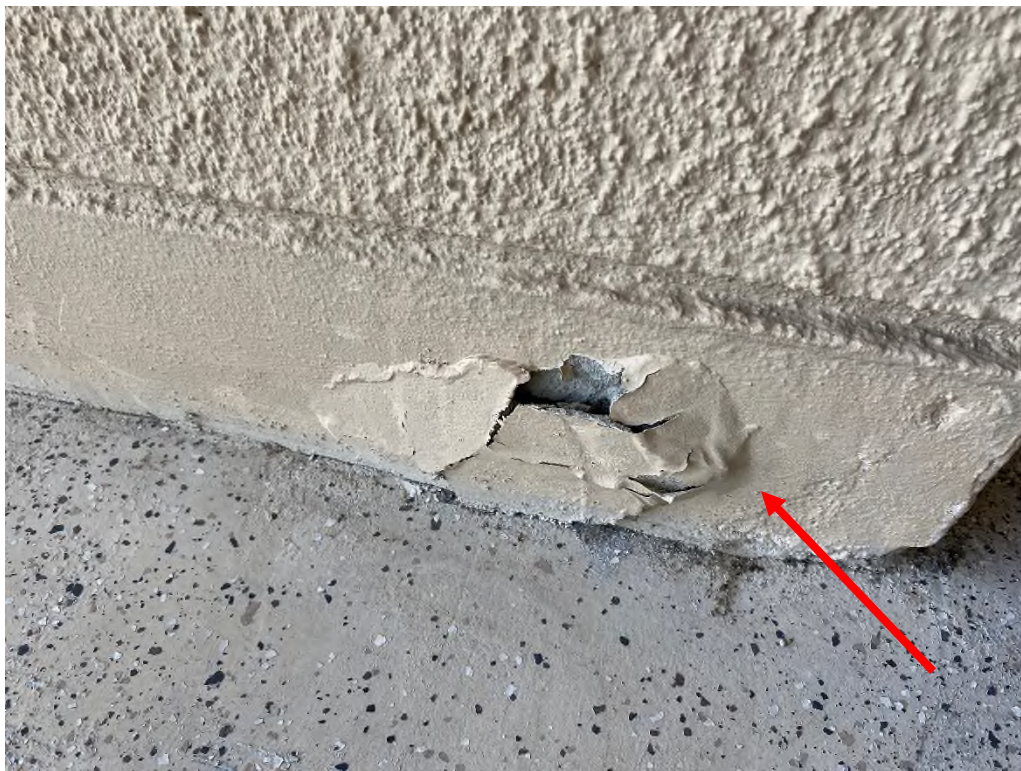
Figure 43 – Delaminated area of wall - Unit 612
