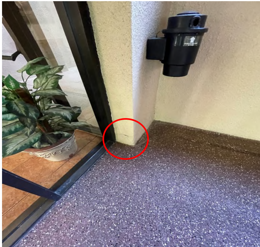
Figure 8 – Identified spalling at column near secure entrance
