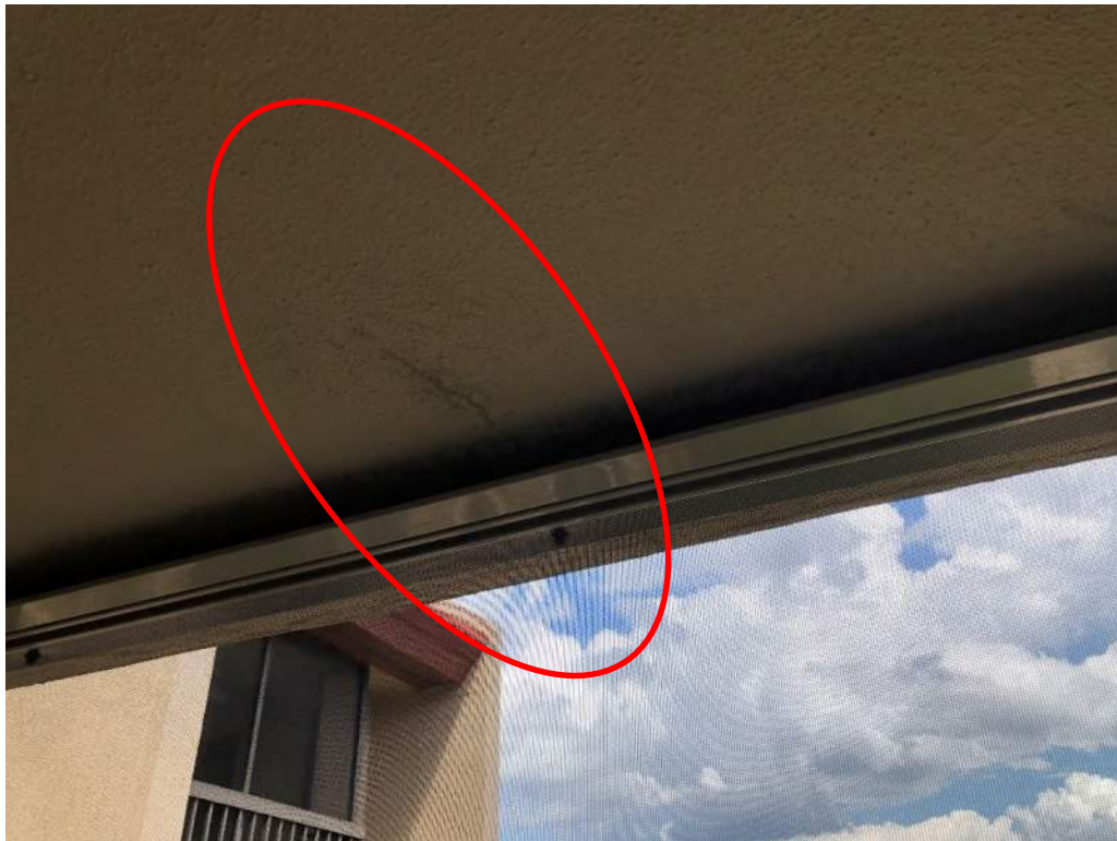
Figure 45 – Spalling located along the overhead floor slab - Unit 516
