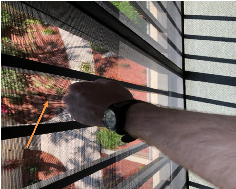
Figure 34 – Picture depicting the relative length between pickets being larger than 4 inches
