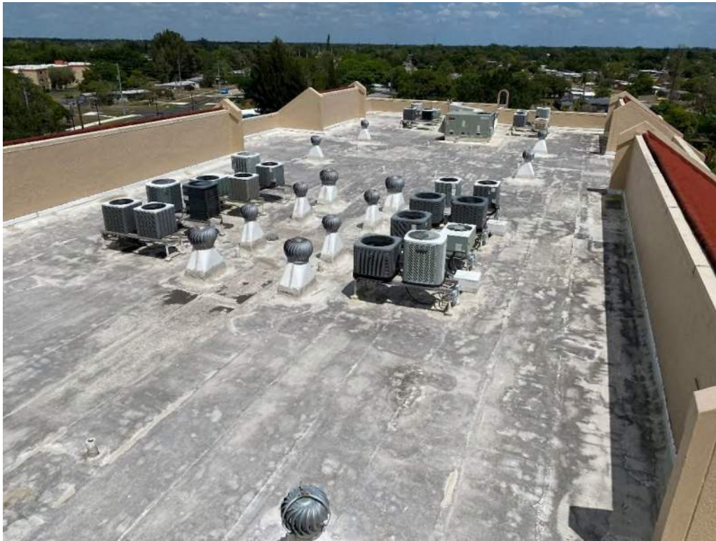
Figure 18 – Overview of the roof
