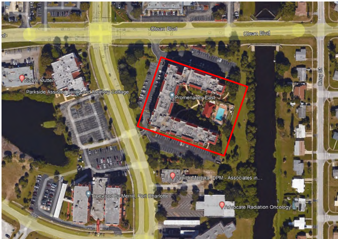
Figure 1 - Aerial View of Promenades East from Google Earth Outlined in Red
